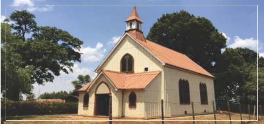
The Watson-Scott Memorial Church was prefabricated in Scotland before being shipped to Kenya
